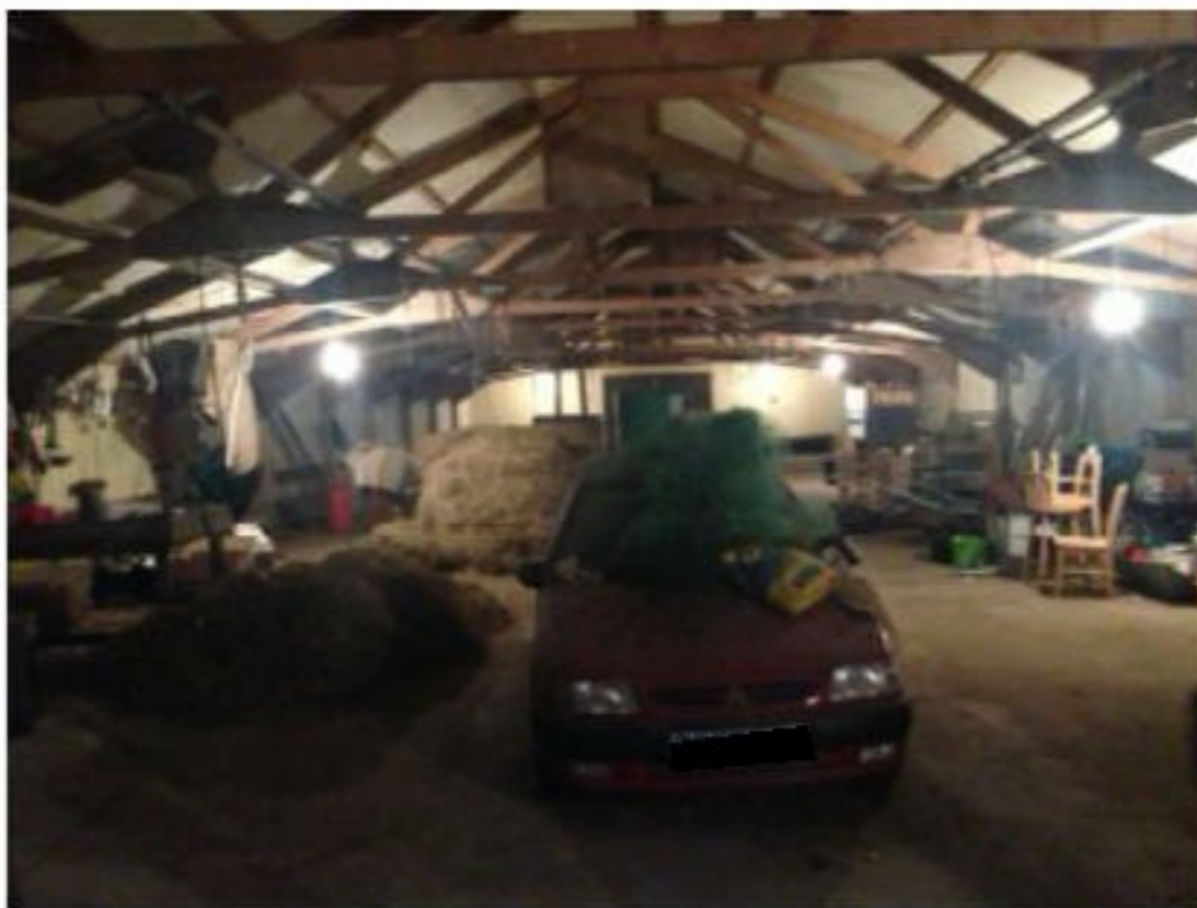
Figure 3. The Shed internal view
