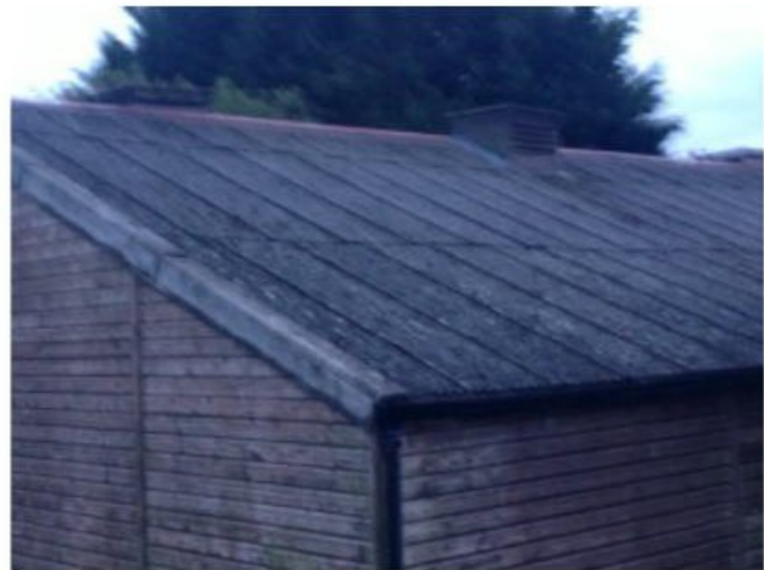
Figure 4. The Shed roof condition
